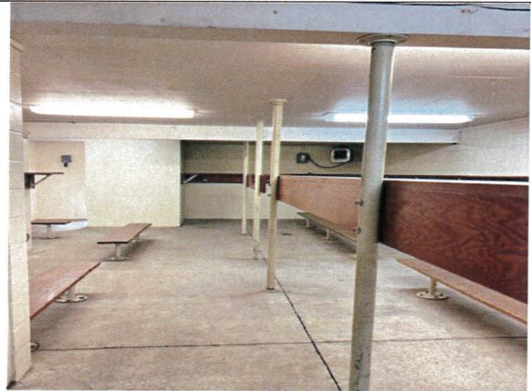
Locker Room/Showers/Bathroom with Wood ceiling, CMU Walls, and Concrete floor. (Negative)
