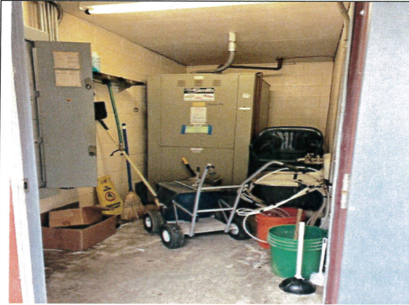
Mechanical Room with Wood ceiling, CMU Walls, and Concrete floor. (Negative)
