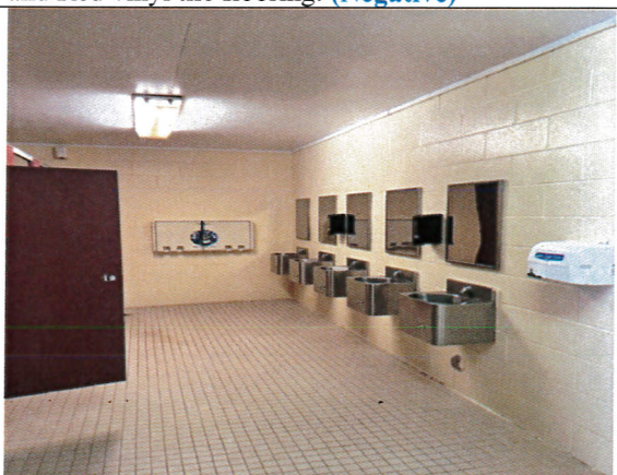
Women's Restroom with Wood ceiling, CMU Walls, and Tile floor. (Negative)
