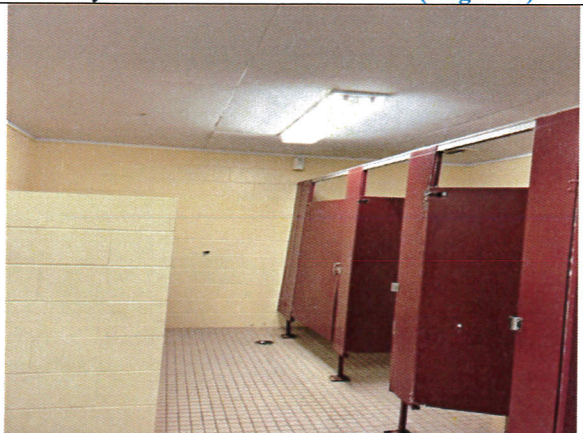
Men's Restroom with Wood ceiling, CMU Walls, and Tile floor. (Negative)
